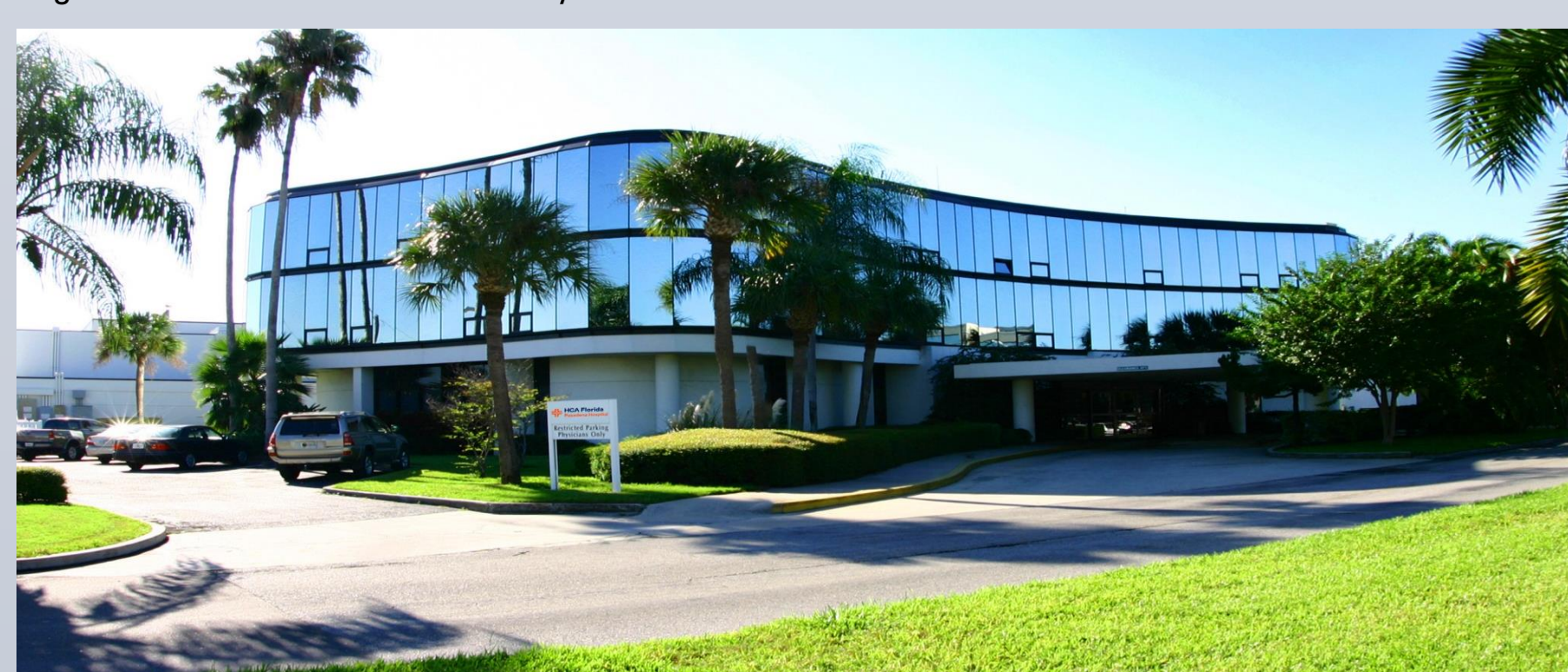
Figure 2. HCA Florida Pasadena Hospital.
